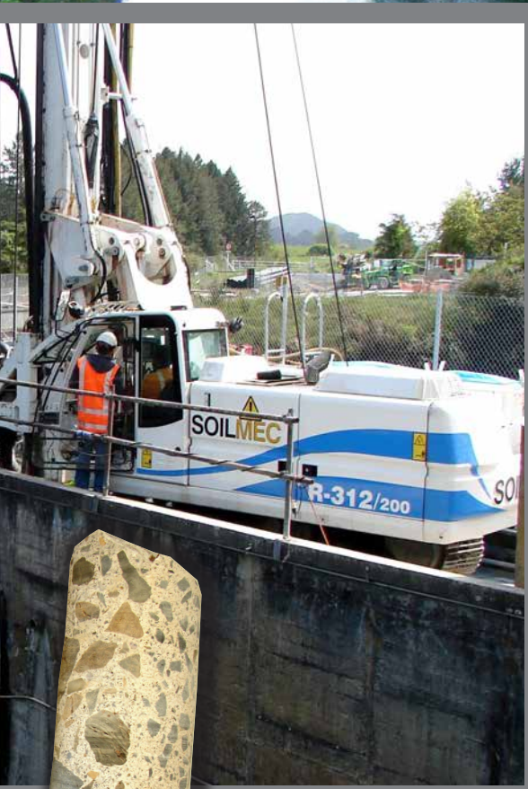
A core sample made from the dam concrete mixed with the 'new' concrete of the panel executed.
